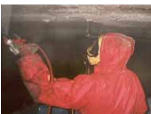
Figure 1.6 Controlled removal of asbestos
