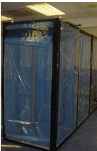
Figure 6.12 Flap arrangements for airlocks
