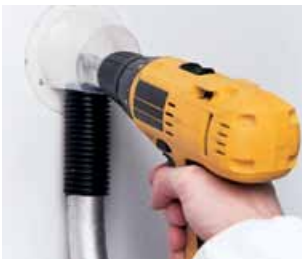
Figure 7.6 Drilling using a low-speed drill with cowl and fitted with LEV
