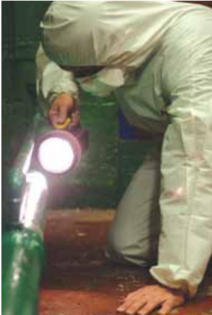
Figure 7.23 Analyst carrying out a visual inspection inside an enclosure
