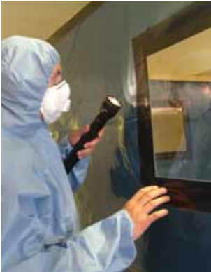
Figure 6.18 A torch being used to find smoke leaks
