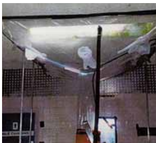
Figure 7.18 A glovebag designed for the removal of sprayed asbestos coatings. Note the gloveports, waste chute and vacuum nozzle used for cleaning and providing slight negative pressure
