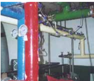
Figure 7.9 Good practice: Wet injection on pipework
