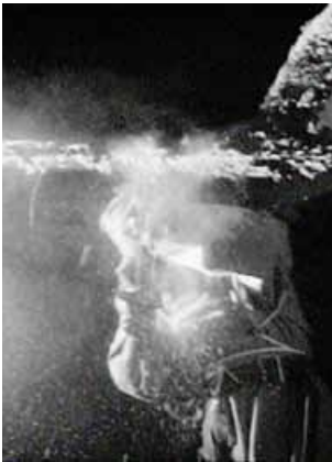
Figure 7.1 Uncontrolled dry stripping
