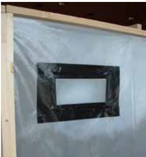
Figure 6.17 An enclosure being smoke tested
