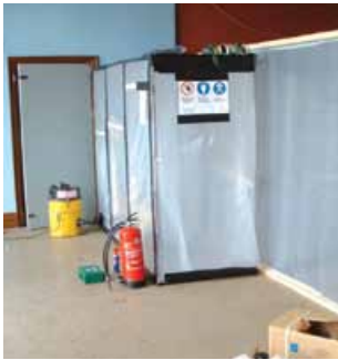
Figure 6.7 An airlock used in transiting
