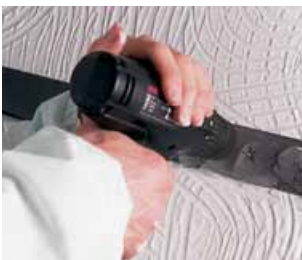
Figure 7.7 Textured coating being drilled through paste
