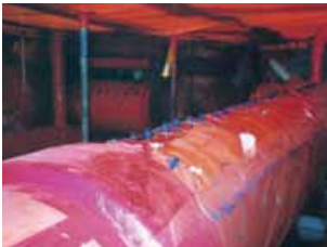
Figure 7.8 Good practice: Wet injection on a large pipe
