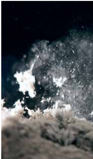
Figure 1.1 Asbestos fibres being released from lagging
