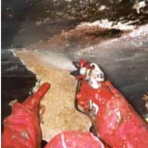
Figure 7.15 Spraying thin coating
