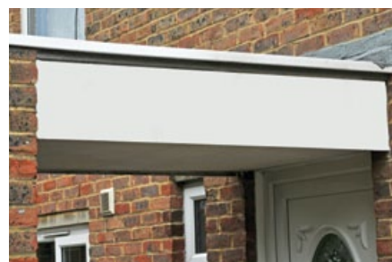
Figure 15 AIB panel in porch
