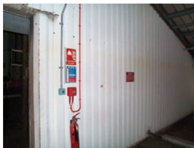
Figure 38 Chrysotile/bitumen coating under metal cladding
