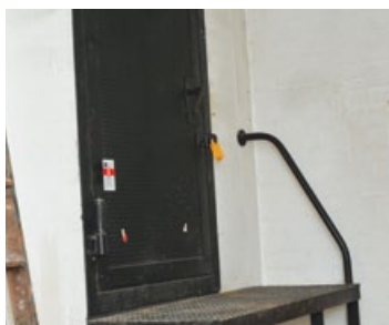
Figure 45 'Durasteel' composite steel and asbestos fire door
