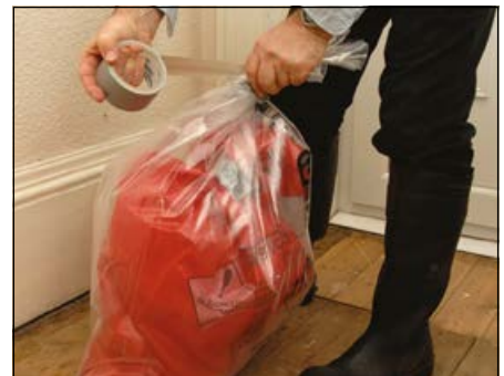
All waste should be double-bagged or double-wrapped in plastic sheeting, with the correct hazard warning signs attached
