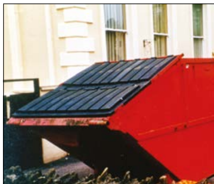
Use a lockable skip for asbestos cement sheet
