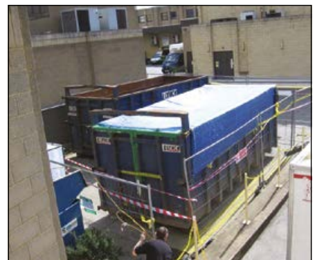
It is not good enough to throw sheeting over a standard skip
