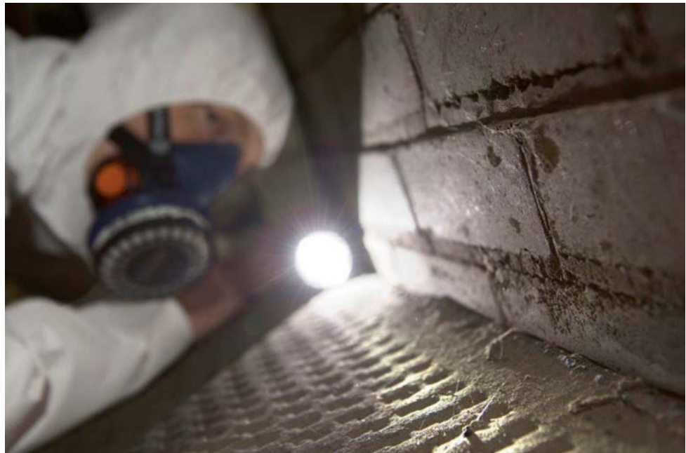
Figure 6.2 Analyst carrying out a detailed visual inspection
