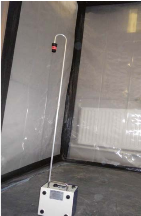
Figure A5.6 Air sampling during clearance
