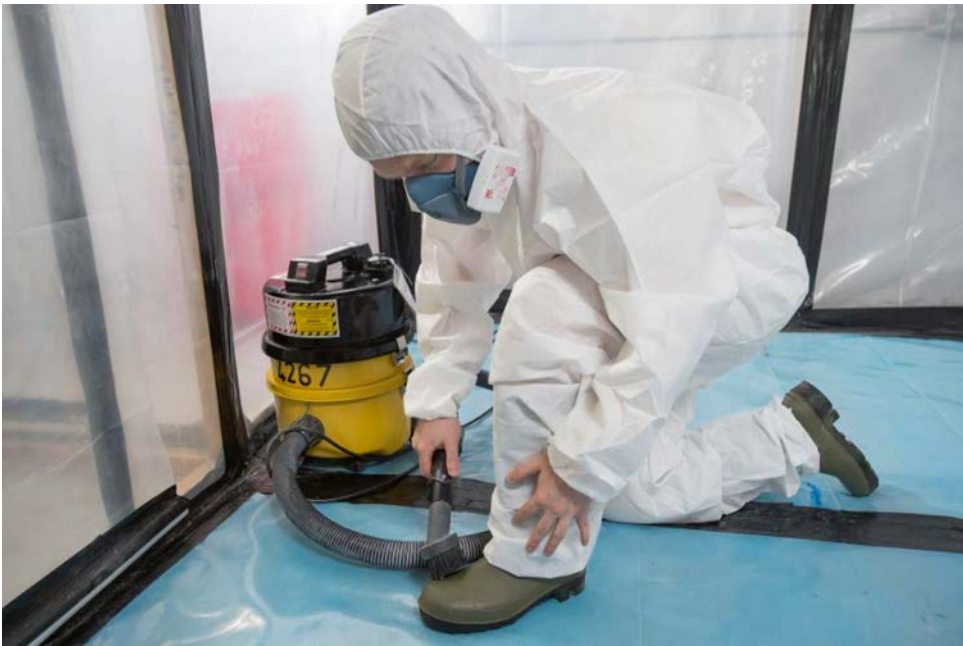
Figure 9.1 Analyst carrying out preliminary decontamination using a Class H vacuum cleaner
