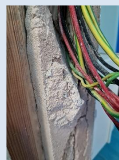
Rough and porous materials where contamination can easily be missed
