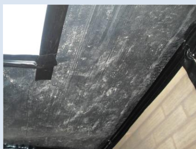
Polythene sheeting including the airlock and baglock
