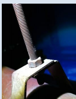
Difficult to clean surfaces like screw threaded bars
