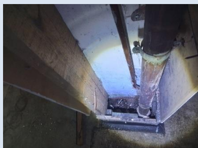
Within fixed boxing which may have become contaminated during removal
