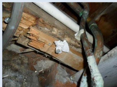
Timber batons where AIB has been attached
