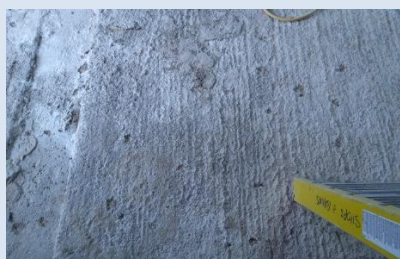
Porous floor or wall surfaces where contamination can collect in the depressions
